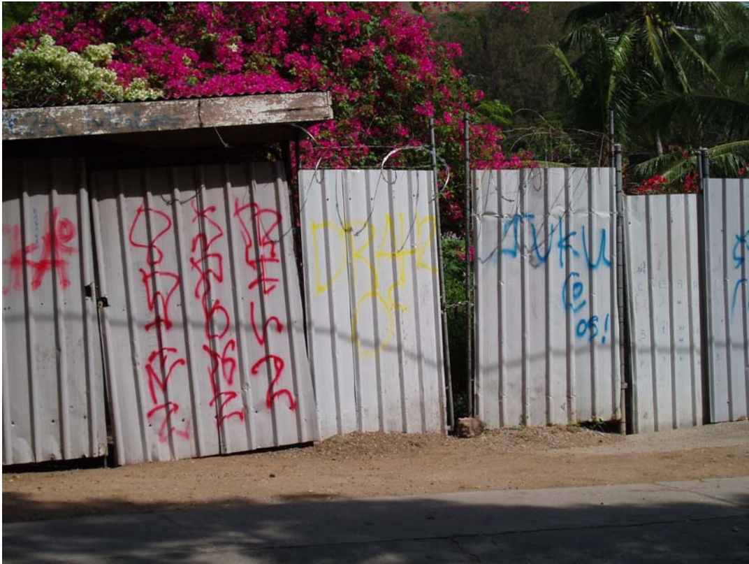
Photo 39a and b: Sheet steel fences offer no resistance to graffiti vandals
