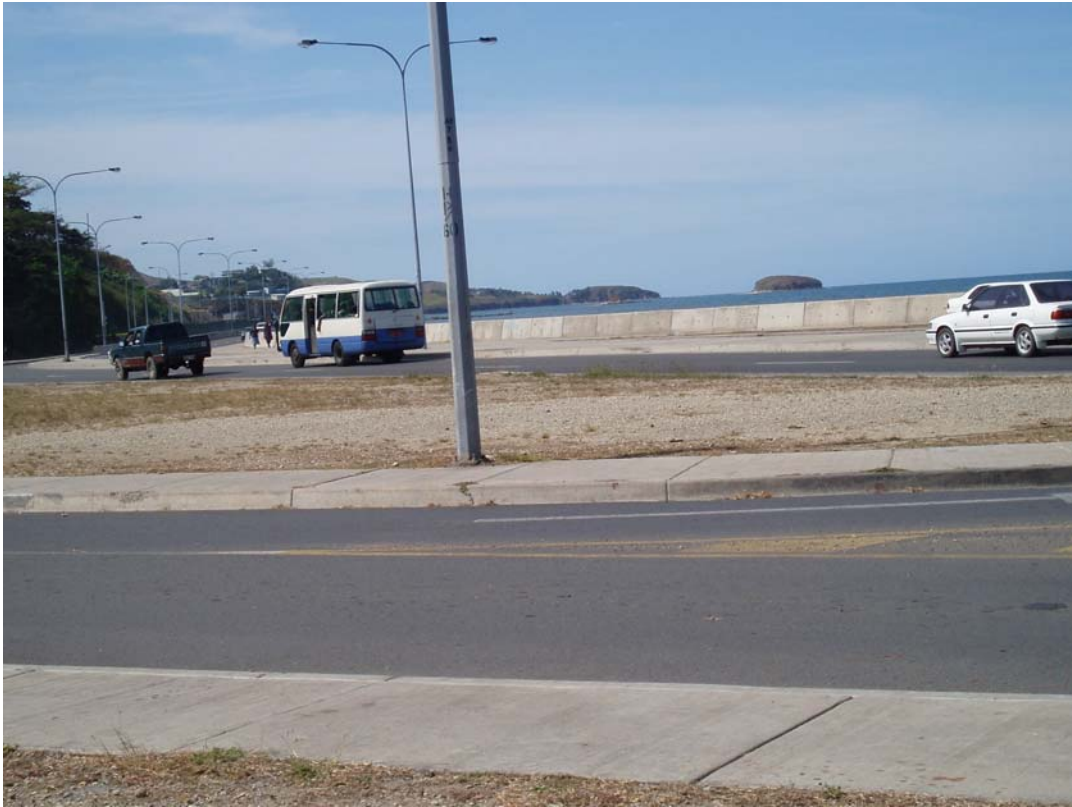
Photo 44: Existing footpath environment lacking normal safety standards
