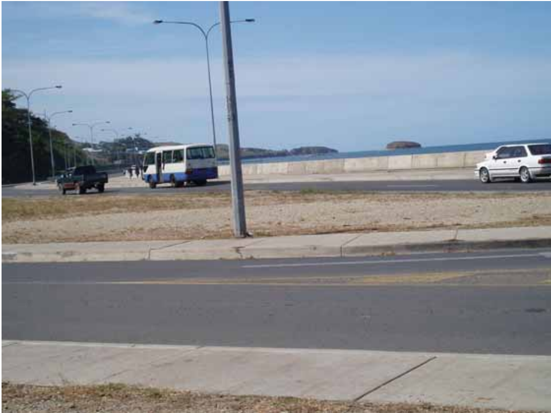
Photo 44: Existing footpath environment lacking normal safety standards
